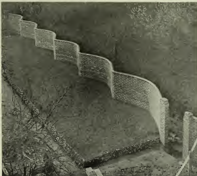
WAVY WALL AT "BELCOMBE," SAXLINGHAM, NEAR NORWICH.
